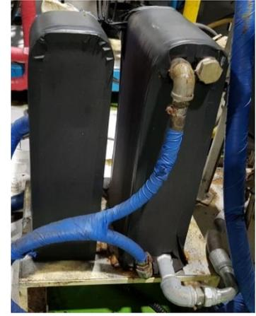
✓ 현장에 설치된 판형 열교환기 Brazing heat exchanger installed in various facilities
