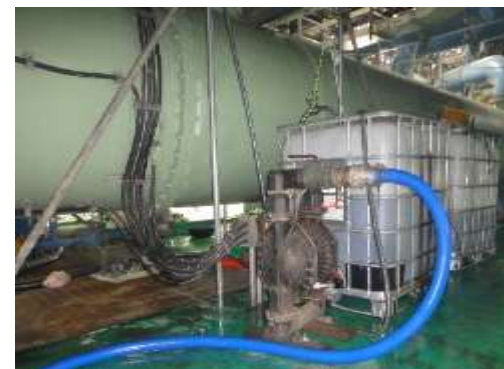
➤ Shell & tube HE Circulation cleaning
