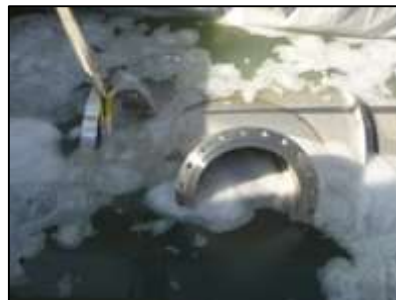
❖ Stainless vessel pickling
