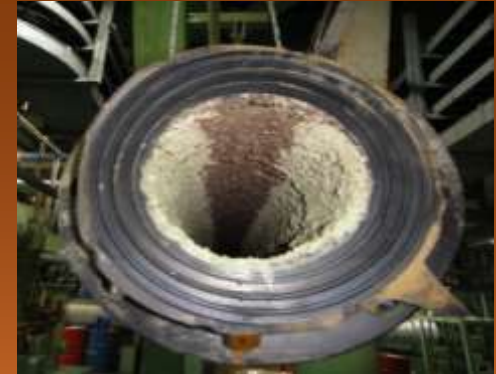
▷ Shellfish inside the sea water cooler tube and pipe
