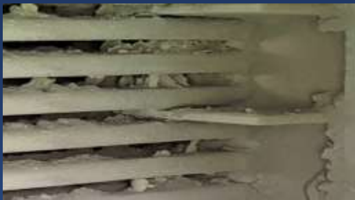
▷ accumulation of ash on furnace inner tube
