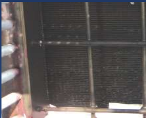
✓ Oil sediments on Compa Block
