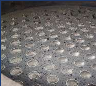
▷ before and after cleaning of scale on tube side
