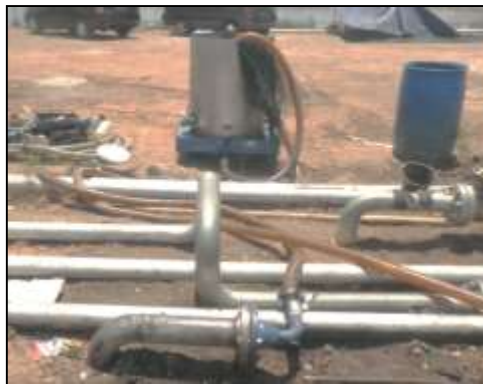
➤ Connection of circulation hose and spool
