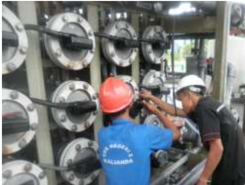
❖ Chlorinator & Desalination Cell cleaning (mineral scale deposits on cell)
