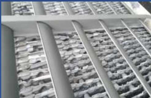
▷ Moss growth of the cooling tower packed bed
