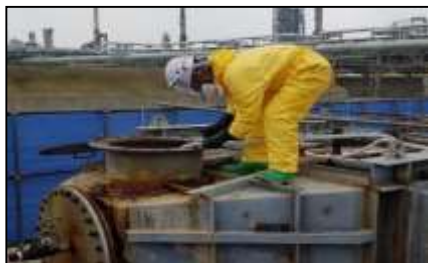
❖ Economizer scale removing
