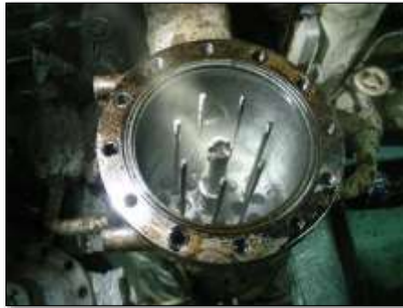
❖ Notch wire filter housing & north type filter elements
