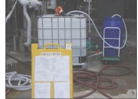
Chemical dosing work
