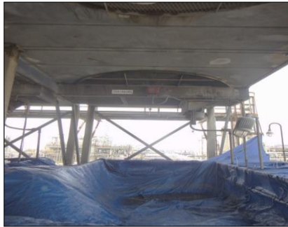
Waterproof canvas and water pool (Preparation for circulating cleaning)
