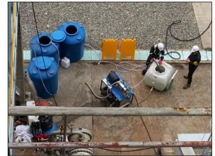
Chemical dosing work
