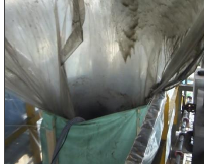
Waterproof canvas and water pool (Preparation for circulating cleaning)
