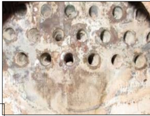
Copper EX / Dip or Circulation 2~4hr / @25~40°C
