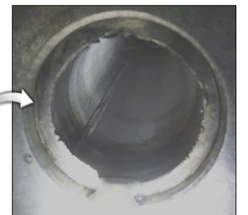
Cooling water piping / Dip or Circulation 2~4hr / @25~40°C
