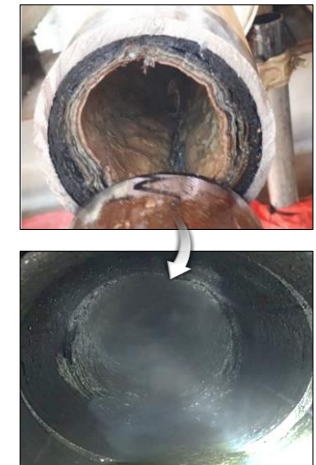
wastewater piping, Struvite Circulation 2~4hr / @25~50°C
