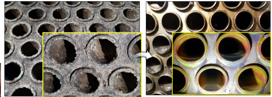
Al-Brass / Dip or Circulation 4~8hr / @25~40°C (power plant CCW, sea water scale)
