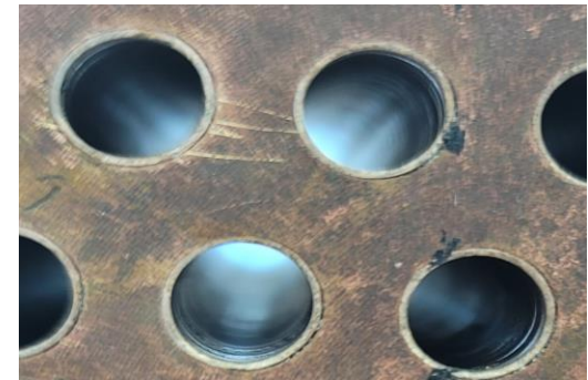
△ after cleaning ( tube inner wall)
