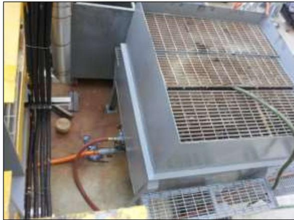
2. Fill up the Hot water to tank @ 65°C
