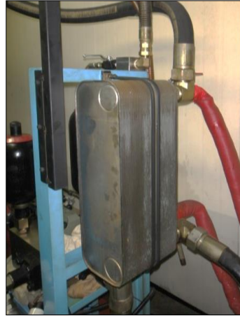
✓ 현장에 설치된 판형 열교환기 Brazing heat exchanger installed in various facilities
