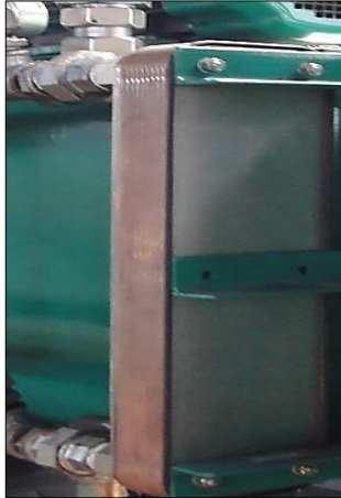
✓ 현장에 설치된 판형 열교환기 Brazing heat exchanger installed in various facilities
